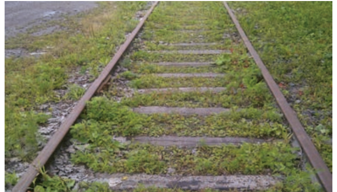
Detail of existing rail lines on Unwin
