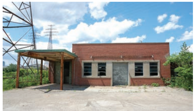
Abandoned structures along the south edge of the Ship Channel
